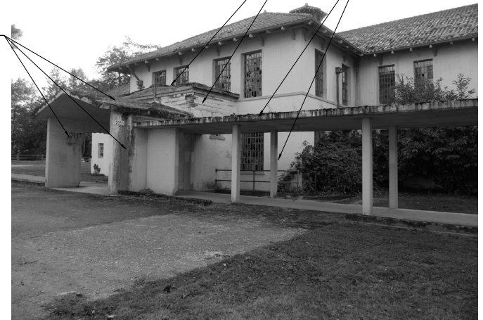
3 Demolition and New Construction at Entry
